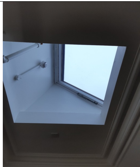
2 nd Floor New Velux Window
