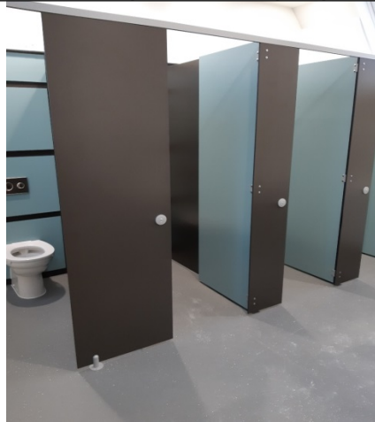
Mezzanine Level Toilets
