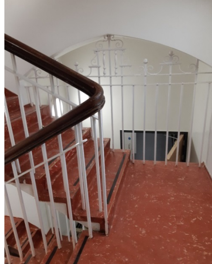
Retained flooring and ironwork to stairwell
