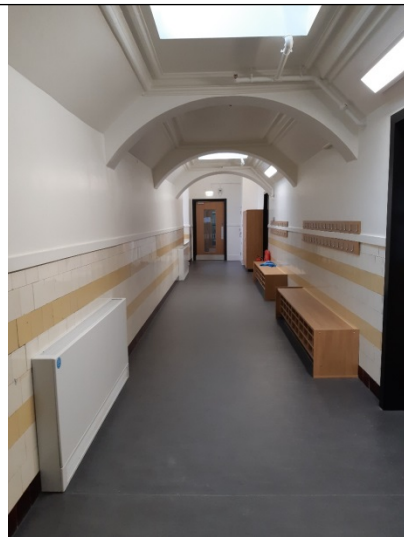
2 nd Floor corridor, retaining existing tiles
