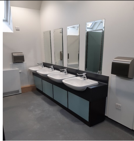
Mezzanine Level Toilets
